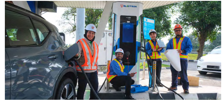
► TNB staff at the TNB Electron Charging Points (DC) at R&R Tapah (Northbound).
