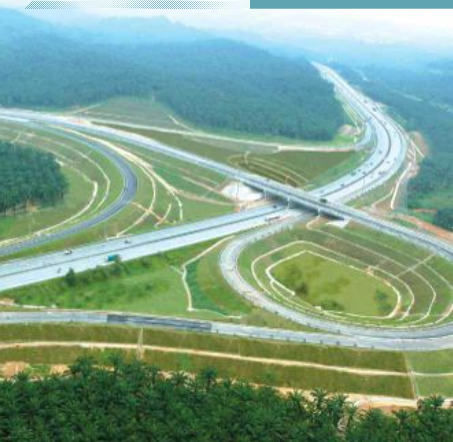
Aerial view of PLUS Malaysia's Sungai Buaya interchange that was opened in January 2014
